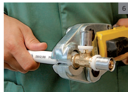
Pressing with TH pressing jaws
