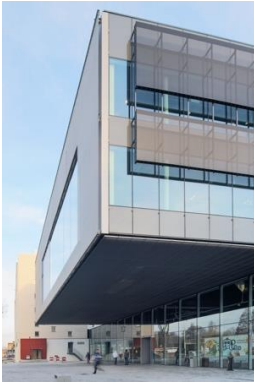
Picture 3: On the upper floors, natural ventilation of the rooms is ensured by VISS parallel vent windows. In this way, the effect of the pure all-glass look can be perfectly maintained.
