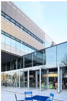
Picture 2: The façade of the "Pulse" university building can be partially opened up so that the cafeteria on the ground floor merges with the square. This is where the VISS system solution, on which the VISS SG pivot doors used are also based, proves its worth.
