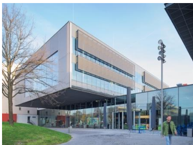
Picture 1: For the façade of the new "Pulse" university building at TU Delft, the architects opted for the VISS SG all-glass façade in structural glazing construction.
